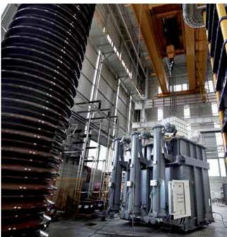
The Electric Arc Furnace and Ladle Furnace Transformers are the key equipment in a steel plant, therefore specific engineering solutions are adopted in order to guarantee over time the best performances under the dielectric, thermal and mechanical stresses which daily involve these transformers.
